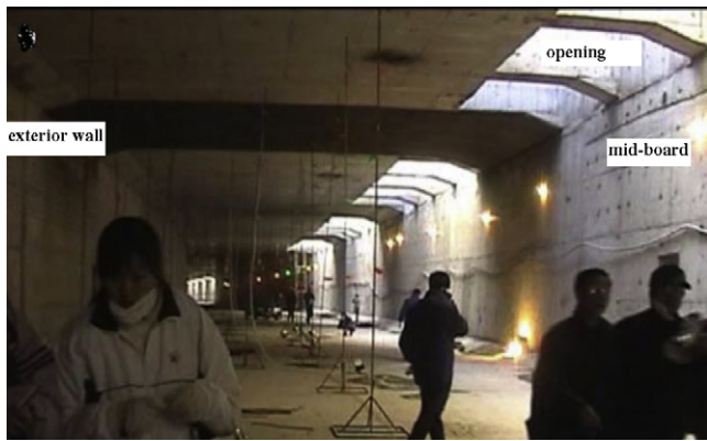
Fig. 1. Interior photograph of tunnel configurations.
